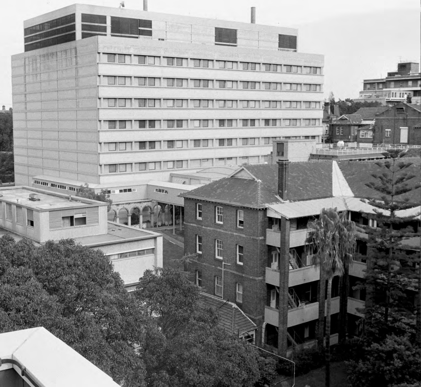
Above: 1998 – the 1910 Nurses' Home extension (right) and Blackburn Pavilion (left) prior to demolition for new Clinical Services Building
